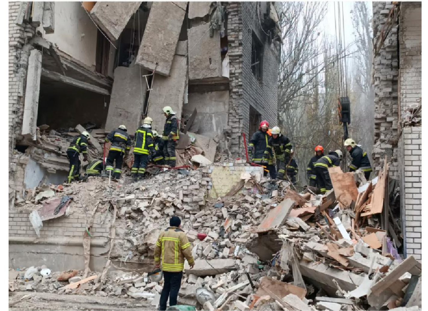
Rescuers work at a site of a residential building heavily damaged by a Russian missile attack, as Russia's attack on Ukraine continues, in Mykolaiv, Ukraine November 11, 2022. REUTERS/Viktoria Lakezina Purchase Licensing Rights
